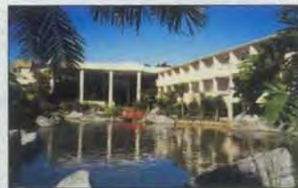
Ramada Resort, North Ryde, Australia. 2,000 sqm. Radcon #7 used to waterproof this lake completely suspended over a car-park.
