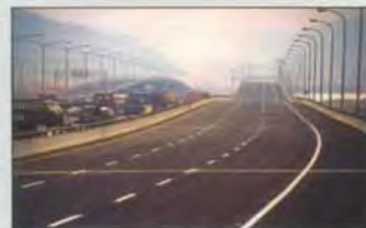
New Taipei Freeway, Taipei, Taiwan. 65,000 sqm. Radcon #7 used to waterproof 4km of raised freeway prior to asphalt topping.
