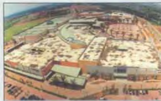
Lippo Karawaci Shopping Centre, Jakarta, Indonesia. 50,000 sqm. Radcon #7 used solely to waterproof this flat concrete roof directly over retail.
