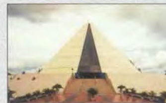
Monument Yogya, Indonesia. Radcon #7 was applied to 5,000 sqm beneath the tiled finish.
