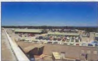
Westfield Market Town, Mt. Druitt, NSW, Australia. 8,700 sqm. Radcon #7 treated to entire car park/rooftop directly over retail area.
