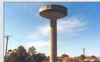
Tempe Water Tower, Sydney, Australia. 1,000 sqm. Radcon #7 used to waterproof the inside of this leaking water tower.
