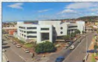
Australian Taxation Office, Wollongong, Australia. 3,500 sqm. Radcon #7 used to waterproof the concrete roof and podium level.
