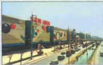
Seacon Square Shopping Centre, Bangkok, Thailand. 50,000 sqm. Radcon #7 applied to entire car park/rooftop directly over retail area.
